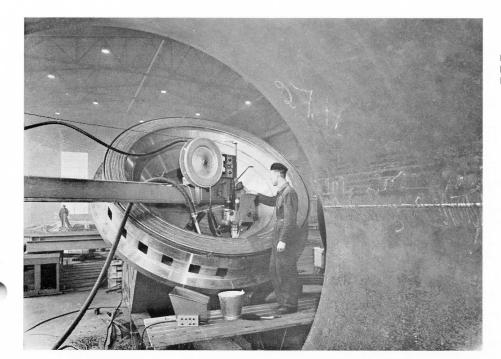
Fig. 7. A layer of stainless steel being welded on the turbine cover by the application of an automatic welding machine.
